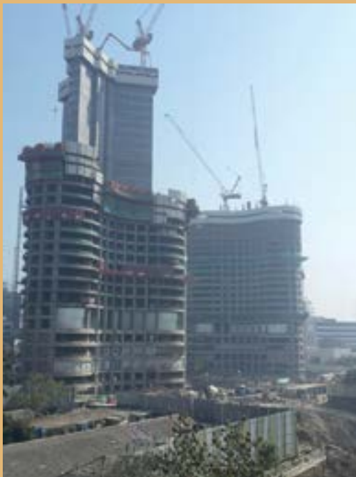
World One under construction in Mumbai (Tallest tower in India)
